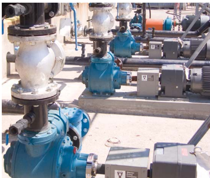
Sliding vane pumps in use at a biodiesel production facility
