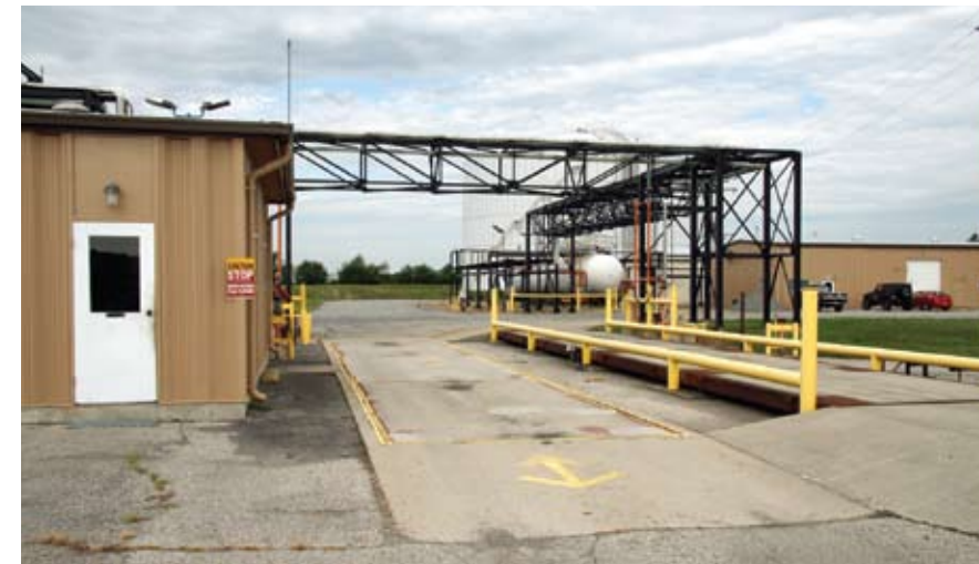
Grammer Industries has its own truck scale at the Van Wert transload location.
