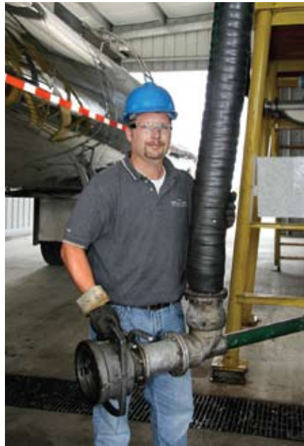
John Whittington holds the OPW loading arm with the OPW bottom-loading coupler at the Morristown transload site.
