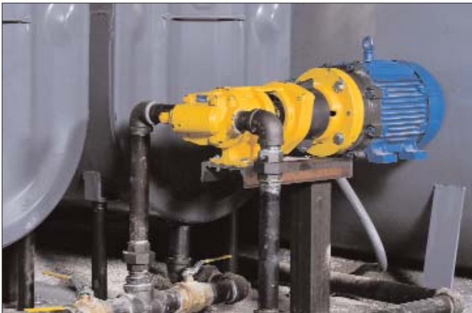
A Blackmer ProVane motor speed sliding vane pump transfers caustic during the production of biodiesel.
