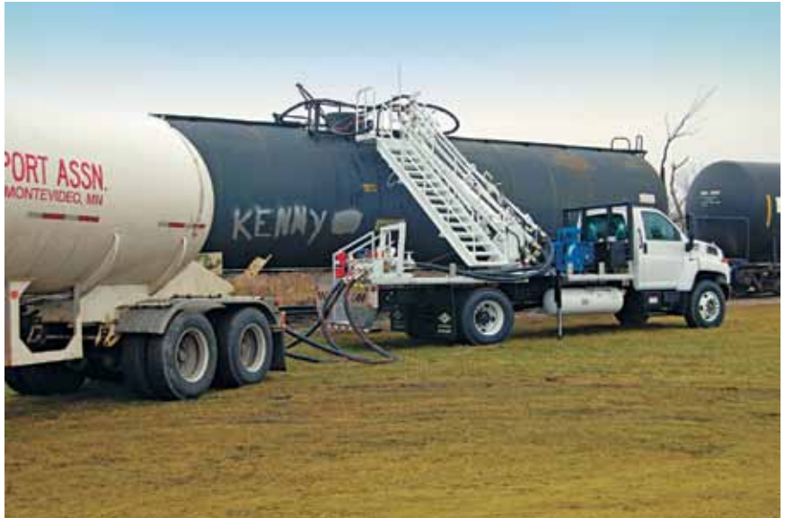
This transloading application features compressors transferring LPG from railcars to transports.
