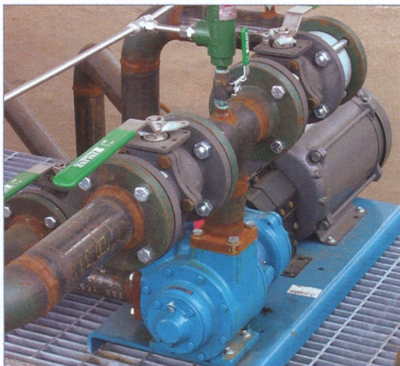
Callahan Chemical selected Blackmer GX Series sliding vane pumps due to their ability to maintain near original volumetric performance levels over a long period of time, high suction lift capabilities and explosion-proof motors.
