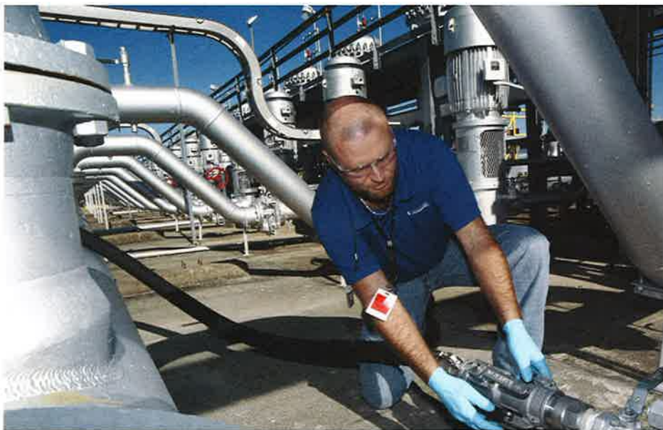
Workers are no longer exposed to everyday spills of product
