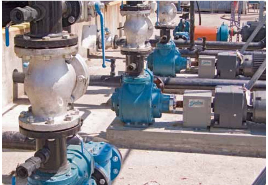
Sliding vane pumps are specifically designed for the needs of terminal operators
